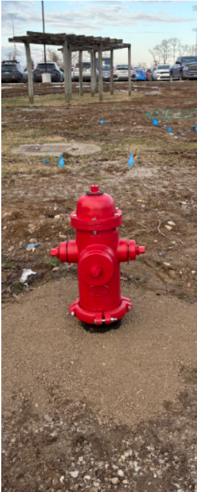
Two newly refurbished fire hydrants.
